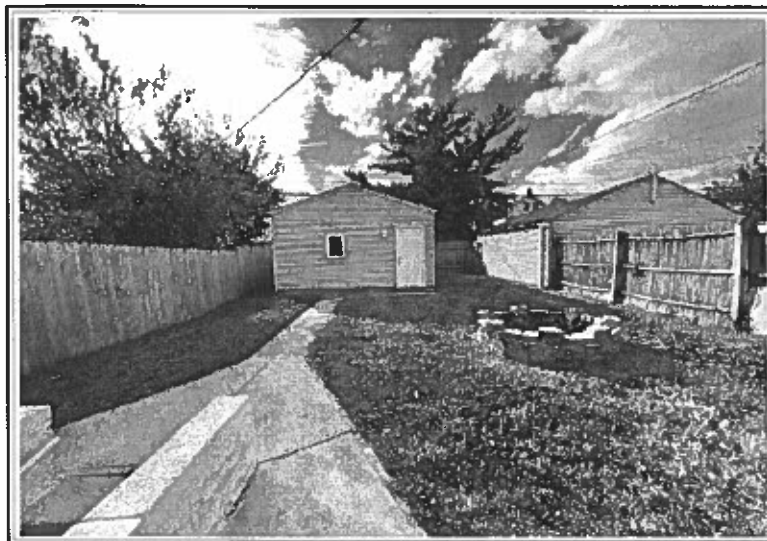
Rear view of the garage
